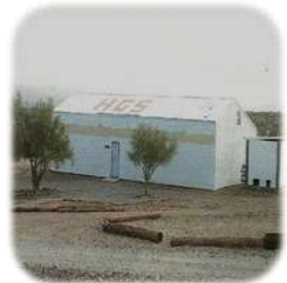
The Pole Barn HGS Equipment Storage
