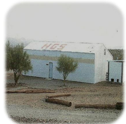
The Pole Barn HGS Equipment Storage
