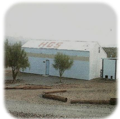
The Pole Barn HGS Equipment Storage
