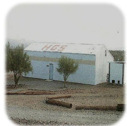
The Pole Barn HGS Equipment Storage
