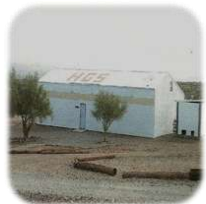
The Pole Barn HGS Equipment Storage
