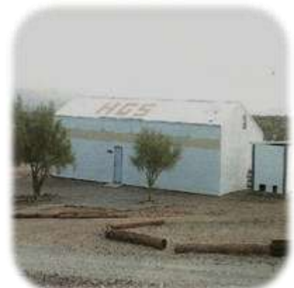
The Pole Barn HGS Equipment Storage
