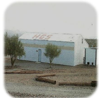
The Pole Barn HGS Equipment Storage
