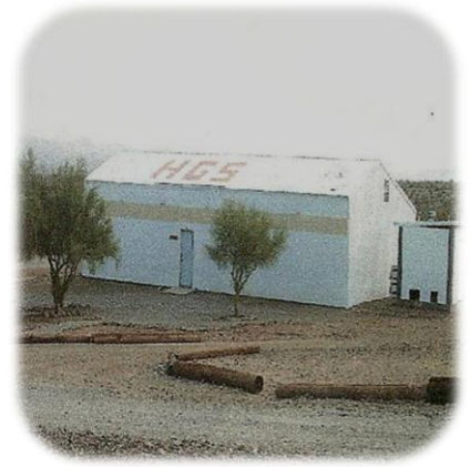
The Pole Barn HGS Equipment Storage
