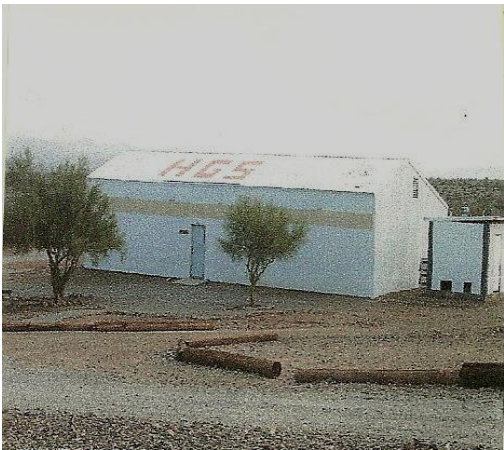
HGS Pole Barn For Equipment Storage
