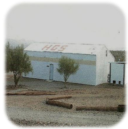
The Pole Barn HGS Equipment Storage
