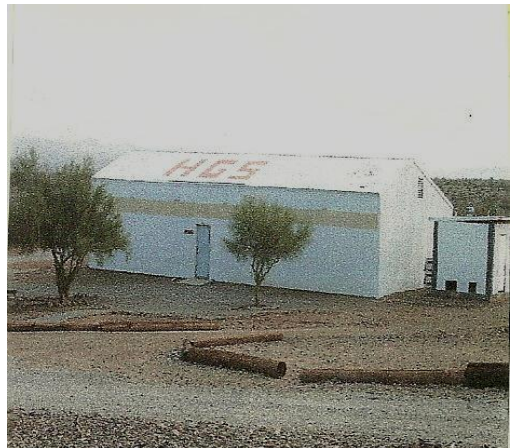
HGS Pole Barn For Equipment Storage
